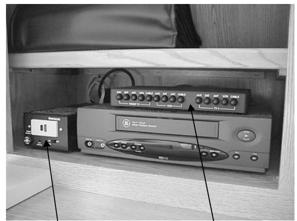
DC/AC Inverter Video Selector System
