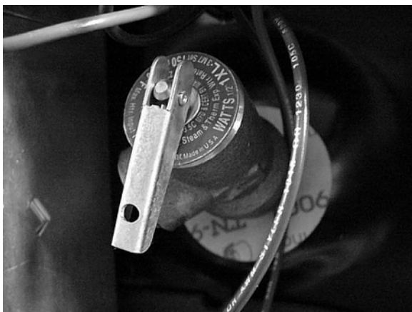
Lift straight out to open P-T valve
