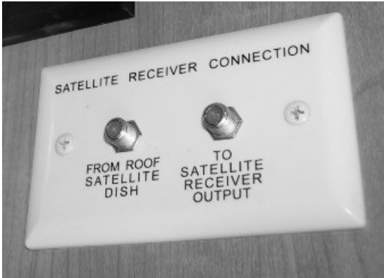
Interior Connection for Satellite Dishes (Located on wall or in cabinet near TV) -Typical View
