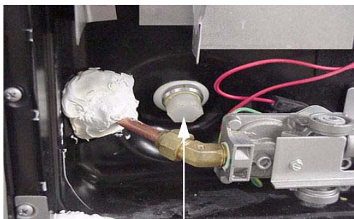
Water Heater Drain Plug (Remove with socket)
