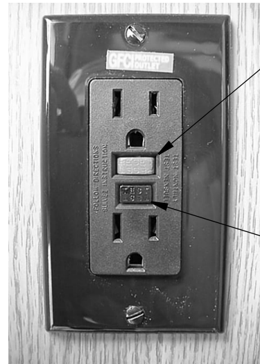
GFCI Outlet (Ground Fault Protector)
