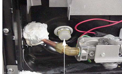
Water Heater Drain Plug (Remove with socket)
