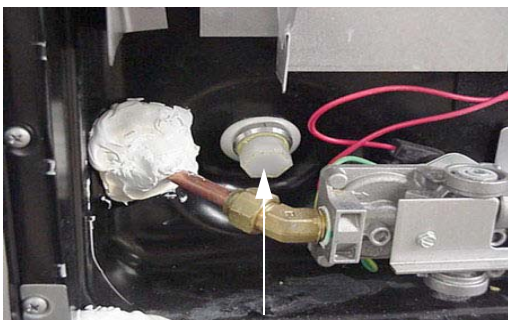
Water Heater Drain Plug (Remove with socket)
