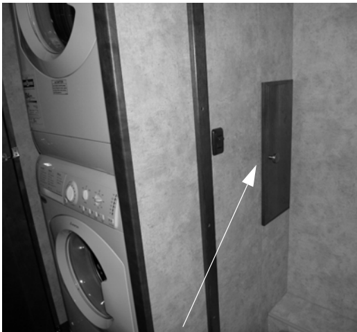
Water Supply Faucets (Located behind access door within the rear wardrobe)
