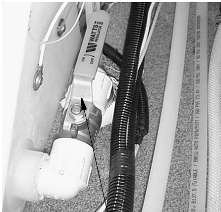
Water Tank Drain Valve (Typical)
