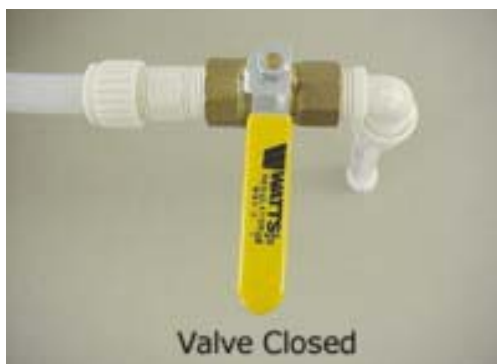
Water Tank Drain Valve (Typical)
