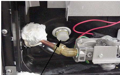
Water Heater Drain Plug (Remove with socket)
