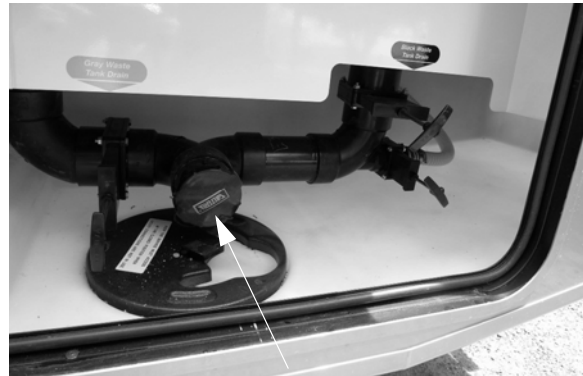
Sewage Drain Outlet (Located in water service center) -Typical View
