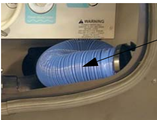
Sewage Drain Hose -Typical View
