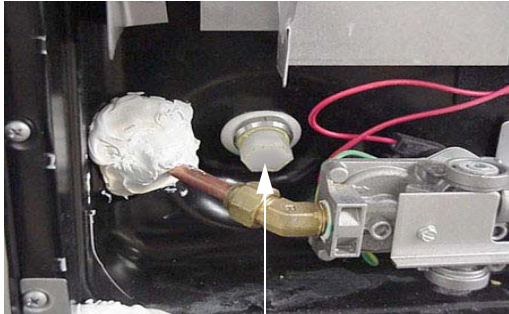
Water Heater Drain Plug (Remove with socket)
