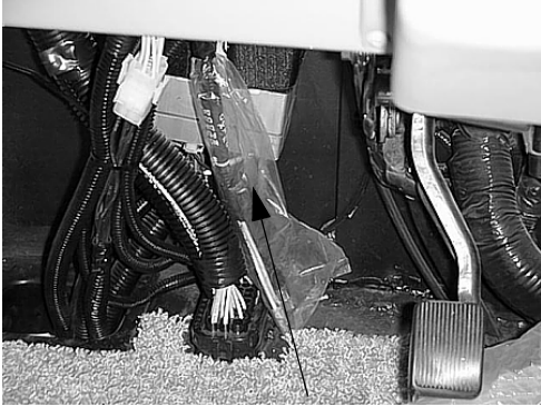
CB Power Wires (in plastic sheath)
