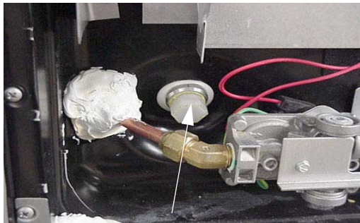
Water Heater Drain Plug (Remove with socket)
