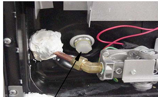
Water Heater Drain Plug (Remove with socket)
