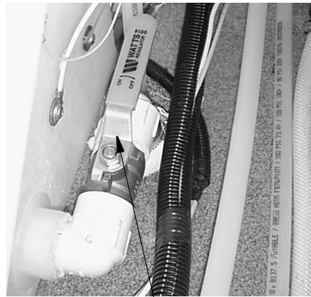
Water Tank Drain Valve -Typical Installation
