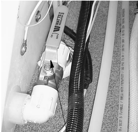
Water Tank Drain Valve (Typical)
