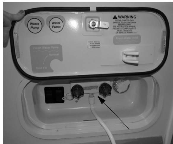
Exterior Shower/Wash Station -Typical View
