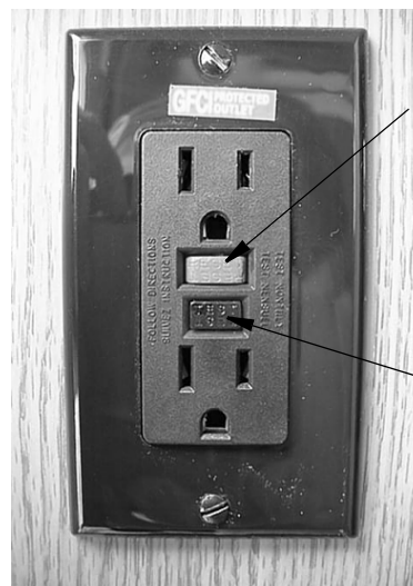
GFCI Outlet (Ground Fault Protector)
