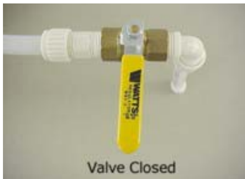
Water Tank Drain Valve (Typical)
