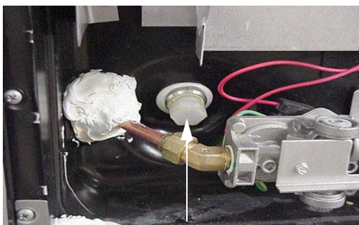
Water Heater Drain Plug (Remove with socket)
