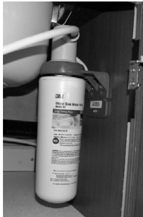
Cold Water/ Ice Maker Filter (Model 34B)
