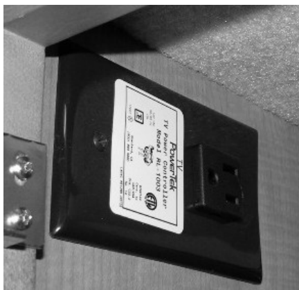
Front TV Ignition Switch Interlock –Typical View
