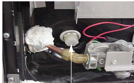
Water Heater Drain Plug (Remove with socket)
