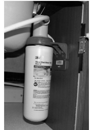
Cold Water/ Ice Maker Filter (Model 34B)
