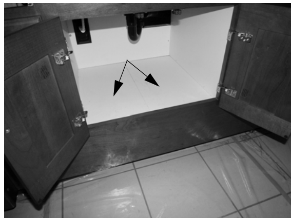
Access Panels (Located beneath lavatory cabinet)
