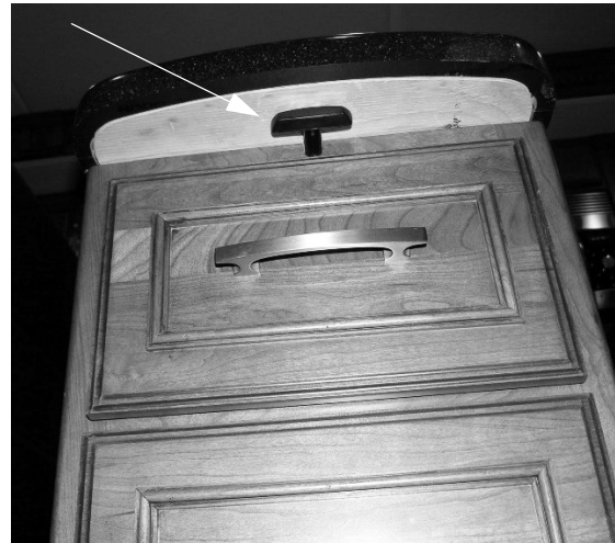
Countertop Extension Release Lever (Located underneath countertop extension lip) -Typical View
