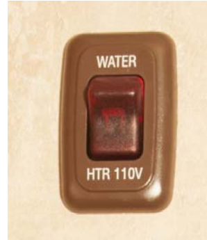
Electric Water Heater Switch (Typically located near Systems Monitor Panel)
