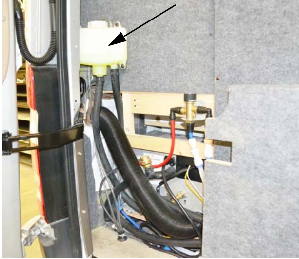
Expansion Fill Tank (Located behind access panel in rear compartment)
