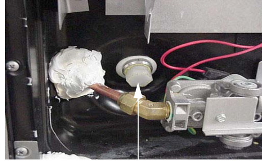
Water Heater Drain Plug (Remove with socket)
