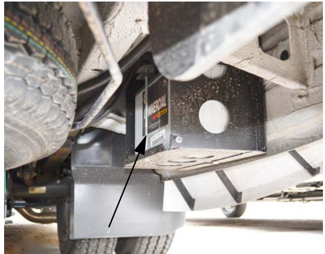
House Battery Access
