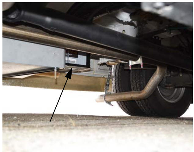
House Battery Access
