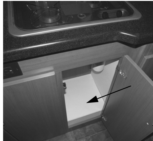
Water Pump (Located beneath removable panel under galley)
