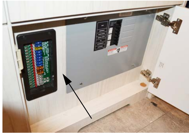
House 12-Volt Fuses (Model 70C) -Typical View
