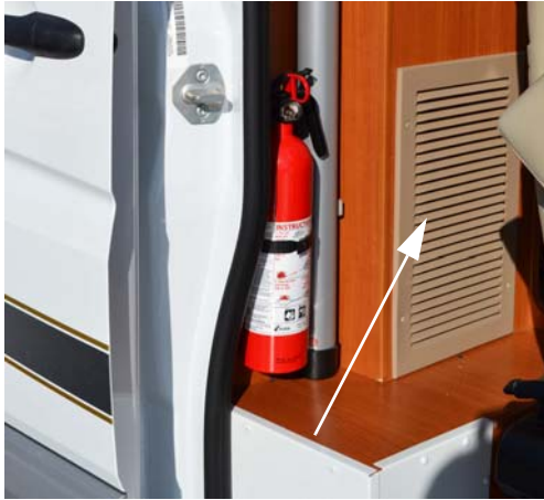
Water Pump (Located behind removable vent on front side of shower cabinet)
