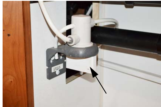
Diverter Plug (installed in filter socket)
