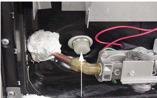
Water Heater Drain Plug (Remove with socket)
