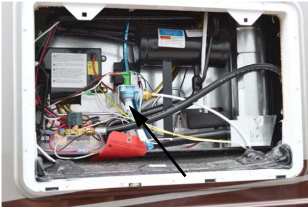
Ice Maker Water Supply Connection -Typical View
