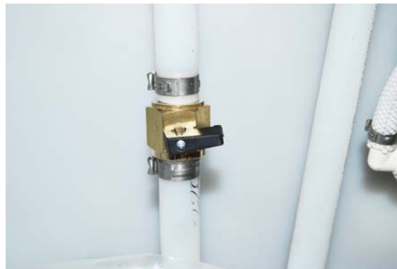
Water Tank Drain Valve -Typical installation shown
