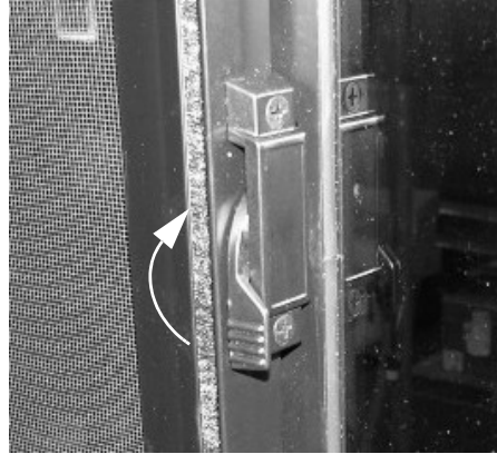
Slider Window Latch (Lift latch UP and slide window open) -Typical View
