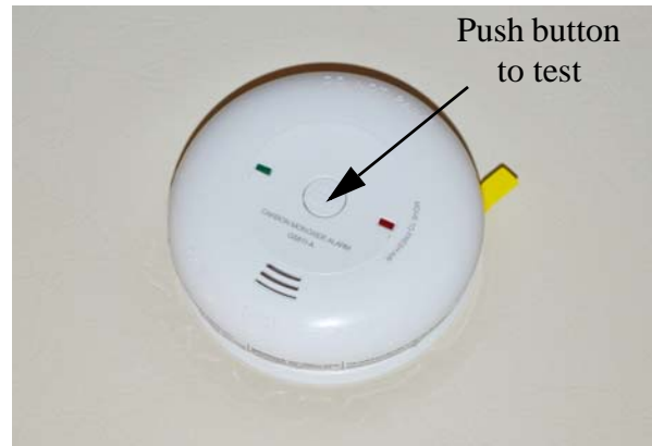
Carbon Monoxide Alarm (9V Battery Required) - Press the Test/Reset button weekly to test
