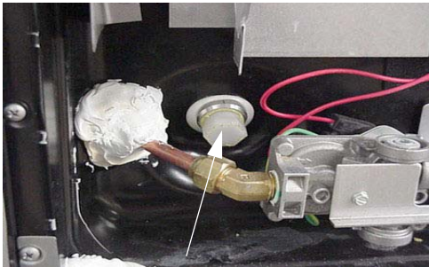
Water Heater Drain Plug (Remove with socket)
