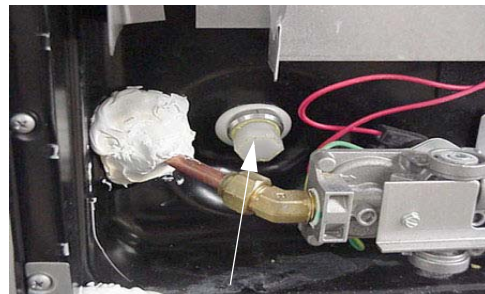
Water Heater Drain Plug (Remove with socket)
