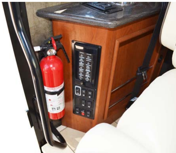
Fire Extinguisher (Located near entrance door) -Typical installation shown
