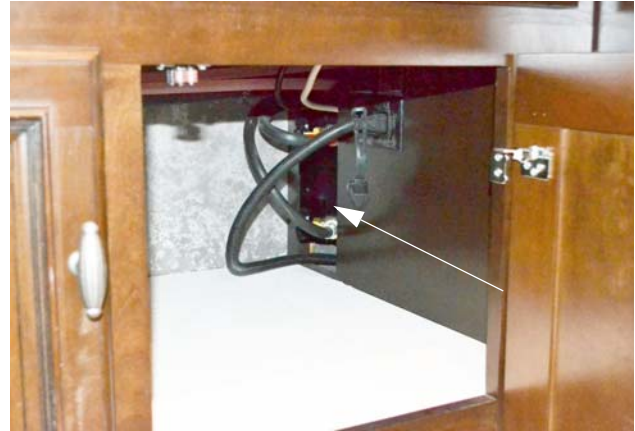
Water Supply Faucets (Located below lavatory cabinet) *Models 42QD
