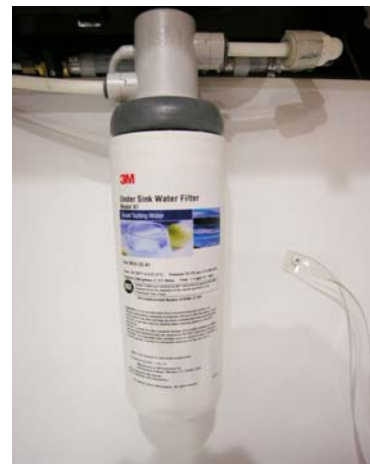
Filtered Cold Water/ Ice Maker Filter (Located below galley sink)
