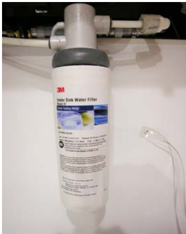
Galley Cold Water Faucet/Ice Maker Filter Assembly (Located below galley sink)
