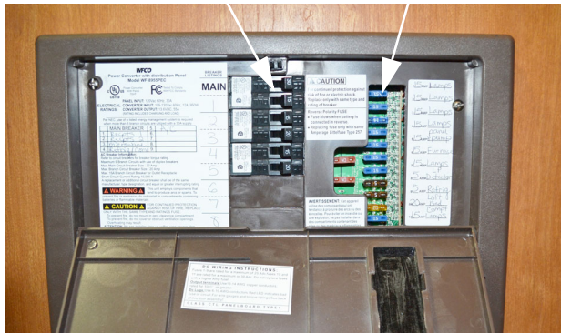
Power Center (Converter) -Typical View
