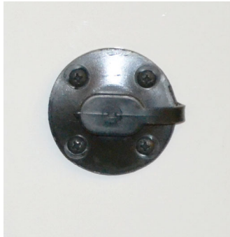
Single Solar Port (Located on an exterior sidewall)
