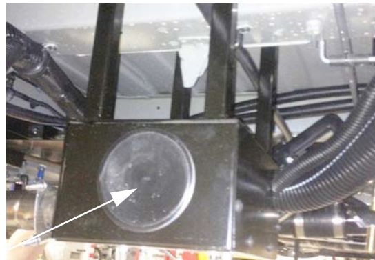
Waste Pump Enclosure (Located beneath motorhome)
