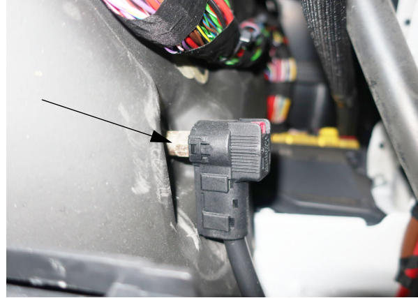
Chassis Battery Connector (Located to the right of the accelerator pedal behind access panel) -Typical View
