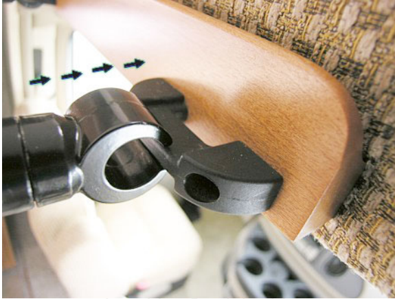
Attaching Bunk Ladder
