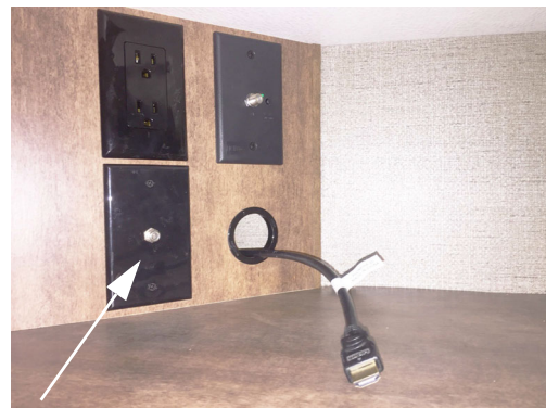
Interior Connection for Satellite Dish -Typical View
