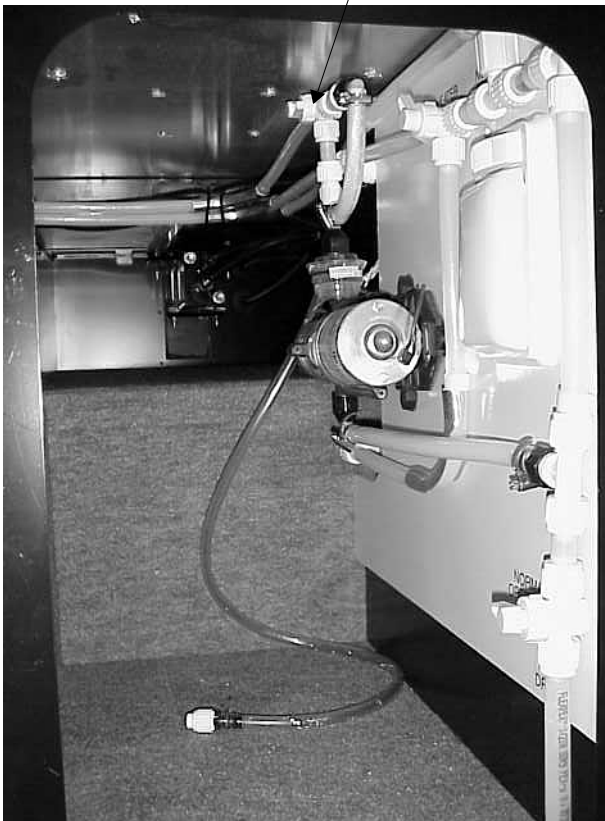
Winterizing Valve & Hose in Right Rear Compartment
