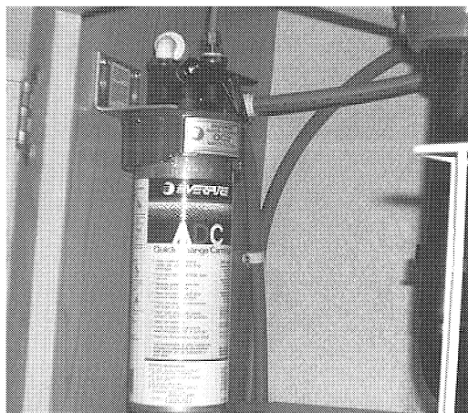
Water Filter Assembly - Below Galley Sink
