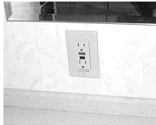
Ground Fault Circuit Interrupter (GFCI)
