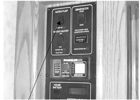
Water Pump Switch
