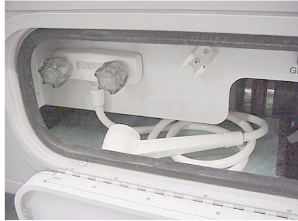
Exterior Shower/Wash Station (Typical)
