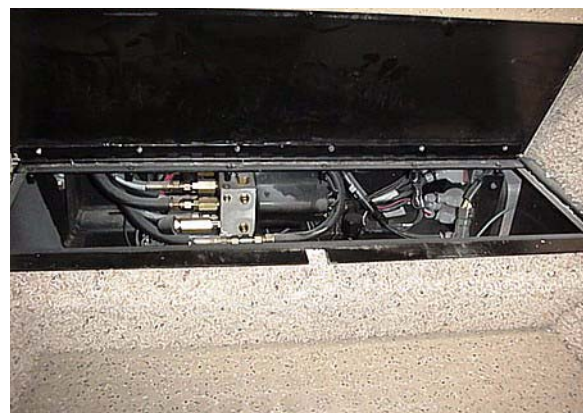
Hydraulic Pump beneath Entry Step
