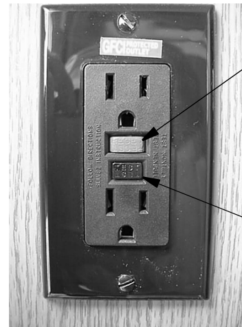
GFCI Outlet (Ground Fault Protector)
