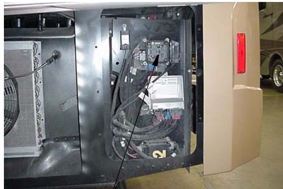
Towing Package fuses are on fuse block
