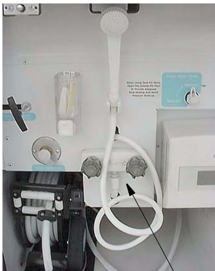
Exterior Wash Station/Shower
