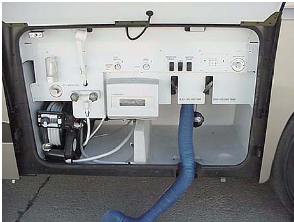
Water Service Center (typical)
