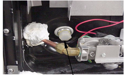
Water Heater Drain Plug Remove with socket.
