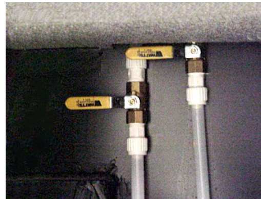
Water Line Drain Valves in Water Center Models 34H & 36G
