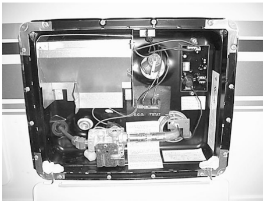
Water Heater Exterior Service Access
