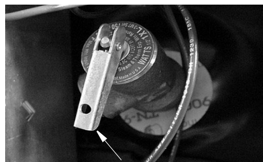
Lift handle only when water heater is cold
