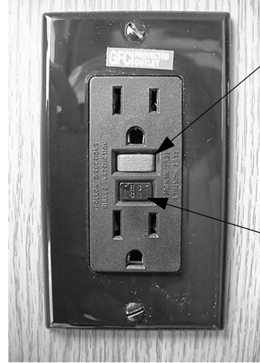
GFCI Outlet (Ground Fault Protector)
