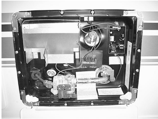
Water Heater Exterior Service Access
