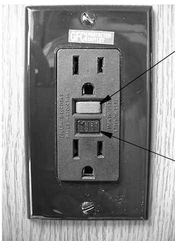
GFCI Outlet (Ground Fault Protector)
