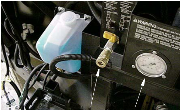
Quick-connect air coupler and air pressure gauge at front end of coach
