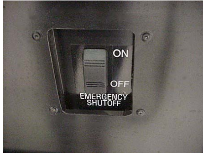
LP Tank Valve in Tank Fill Compartment
