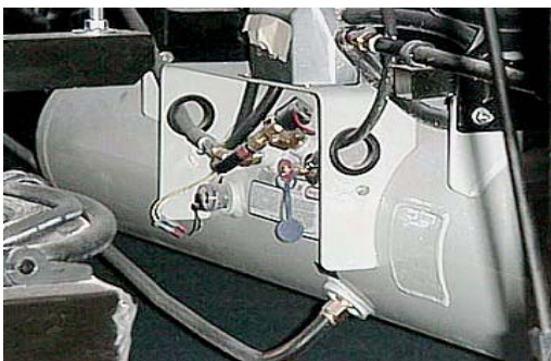
LP Gas Tank behind slideout room
