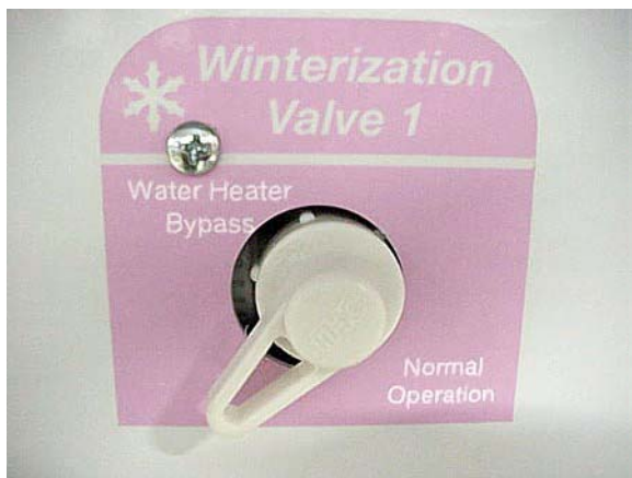
Water Heater By-Pass Valve
