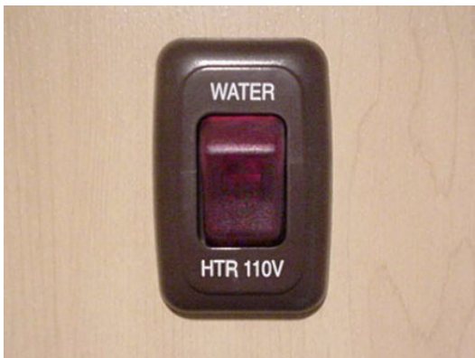
Electric Water Heater Switch (Typical) Located Near Systems Monitor Panel
