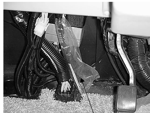
CB Power Wires (in plastic sheath)
