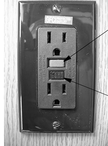
GFCI Outlet (Ground Fault Protector)
