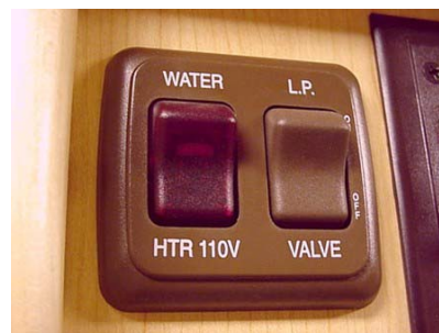
Main Tank Valve on OnePlace Panel
