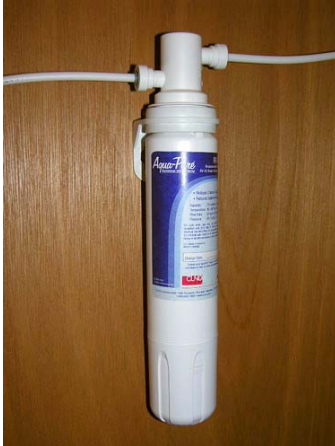
Water Filter Assembly (Located below Galley Sink)
