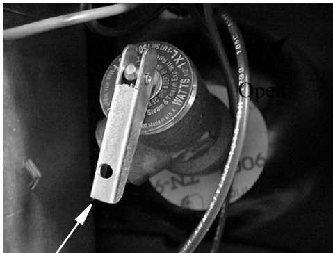
Lift handle straight out to open P-T valve when water heater is cold *
