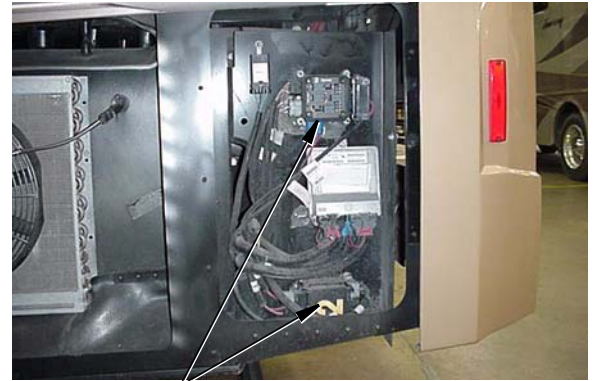
Chassis Fuse & Relay Blocks
