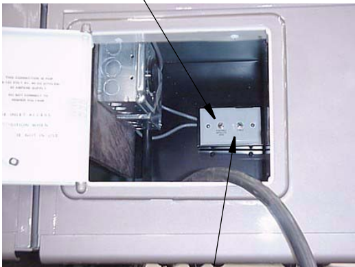
Portable Satellite Dish Hook-up in Shoreline Compartment
