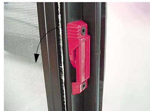
Pull latch outward to slide window open
