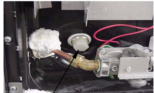
Water Heater Drain Plug Remove with socket.
