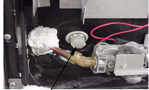
Water Heater Drain Plug Remove with socket.
