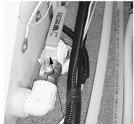
Water Tank Drain Valve (Typical)
