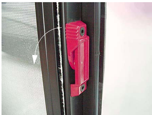
Pull latch outward to slide window open
