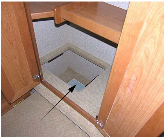
AC/Furnace Filter Access *MODELS 40BD and 40WD (Located under wardrobe floor panel) -Typical View Filter Size: 14" x 20" x 1"
