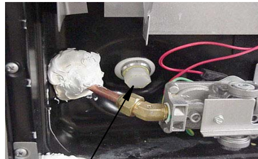
Water Heater Drain Plug (Remove with socket)
