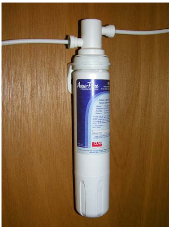
Water Filter Assembly (Located below galley sink)
