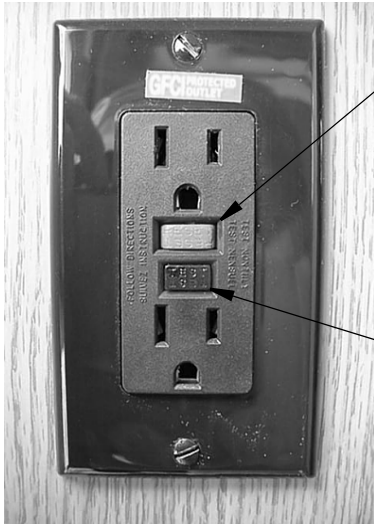
GFCI Outlet (Ground Fault Protector)
