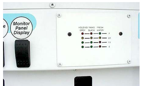
Water Center Tank Level Monitor -Typical View
