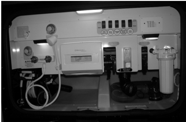
Water Service Center - Typical View
