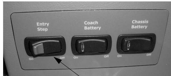
Entry Step Switch (Located near the entrance door) -Typical View
