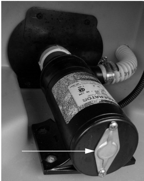
Waste Pump Manual Access (Remove end cap to manually turn pump shaft) -Typical View
