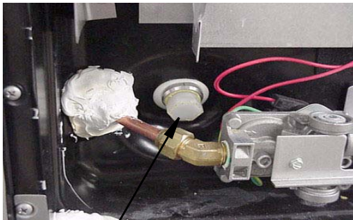
Water Heater Drain Plug (Remove with socket)
