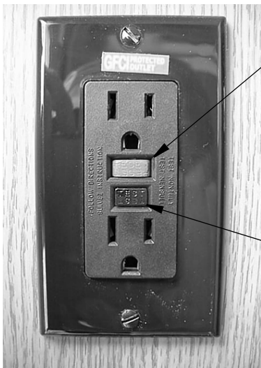
GFCI Outlet (Ground Fault Protector)
