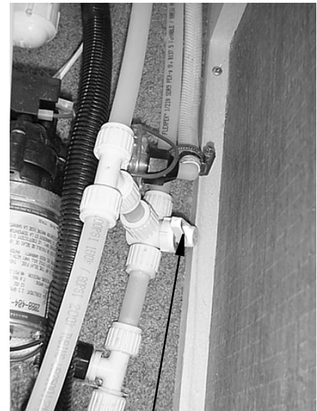
Waterline Drain Valve (Typical)
