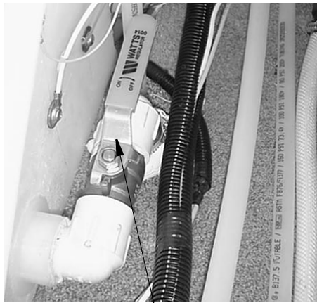
Water Tank Drain Valve (Typical)
