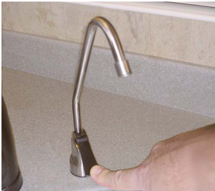
Filtered Water Faucet -Typical View
