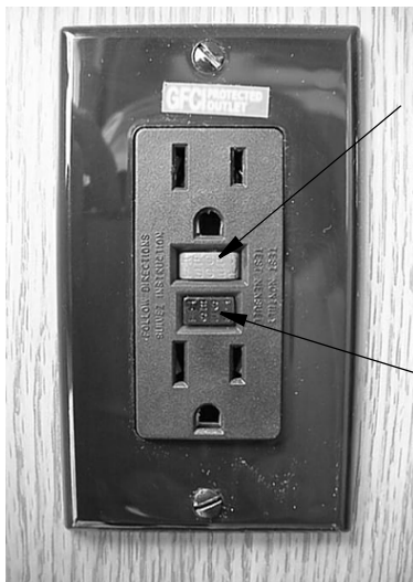
GFCI Outlet (Ground Fault Protector)
