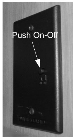
TV Signal Amplifier Switch (Located inside overhead cabinet near TV) -Typical View
