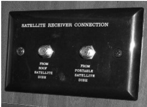
Interior Connection for Satellite Dishes (Located in cabinet near TV) -Typical View
