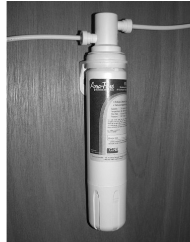
Ice Maker Filter Assembly (Located below galley sink) -Typical Installation
