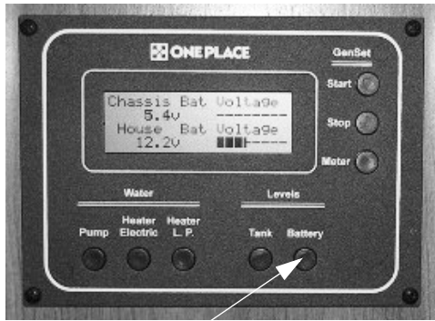
Battery Levels Switch
