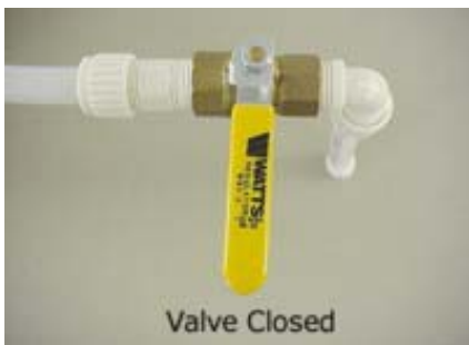
Water Tank Drain Valve -Typical installation shown
