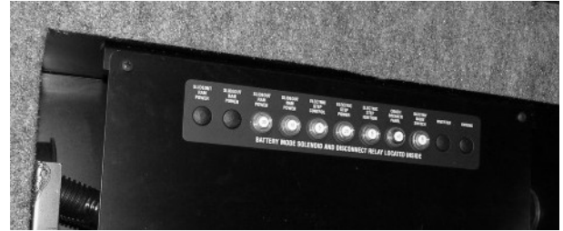
Automotive Chassis and House 12-Volt Circuit Breakers (Located inside passenger compartment) -Typical View
