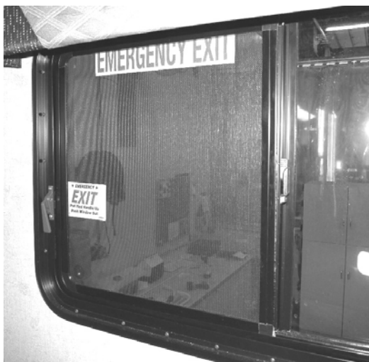
Bedroom Escape Window (Lift both red safety latches UP and push window OUT for emergency exit) -Typical View
