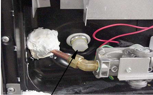
Water Heater Drain Plug (Remove with socket)
