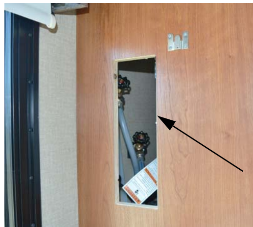
Water Supply Faucets (Located behind picture rear of washer/dryer) *Model 36G
