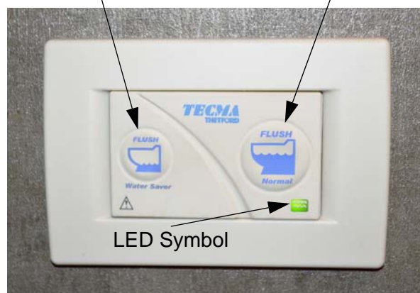
Wall Switch/Controller (Located on wall near toilet)
