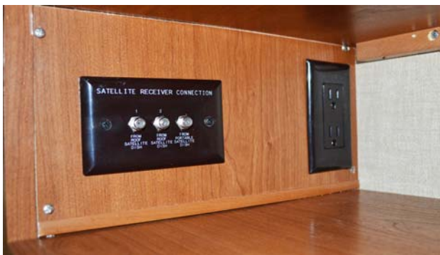
Interior Satellite Dish Connections (Located in the entertainment center cabinet) -Typical View
