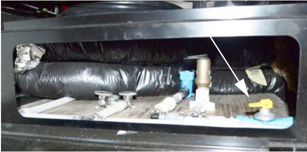
Water Heater Drain Valve (See “Water System Drain Valve Locations” chart at the end of this section for location on your model) *Model 70X shown
