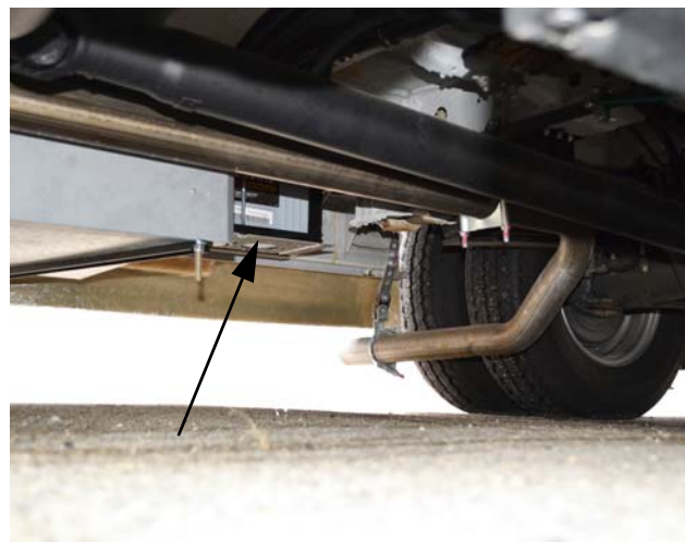
House Battery Access
