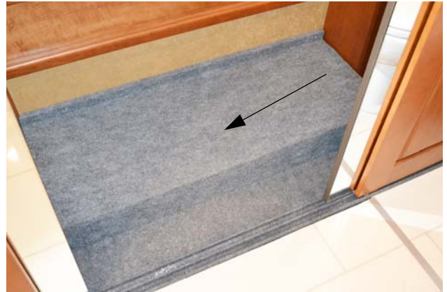
Access Panel (Located on bathroom wardrobe floor)
