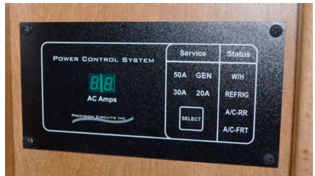
PCS Display Panel (Located near monitor panel) -Typical View
