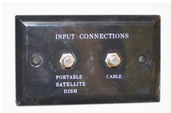
Satellite Dish and Cable TV Connections (Located in utility compartment or water service center) -Typical View
