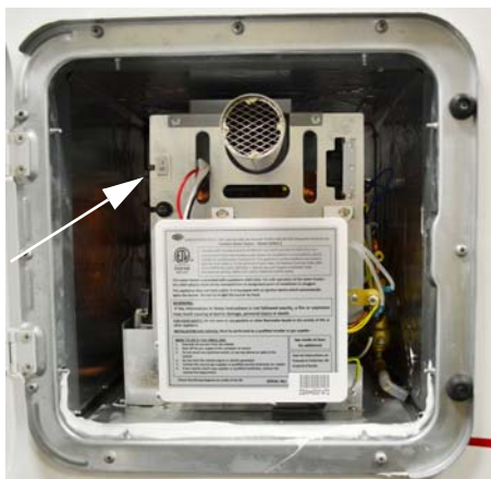
Water Heater Power Switch (Located inside water heater door)
