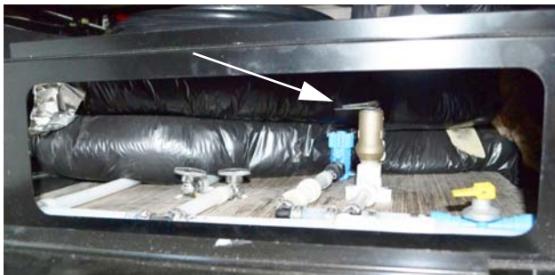
Pressure Temperature Relief Valve
