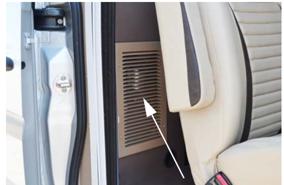
Water Pump (Located behind removable vent on front side of shower cabinet)
