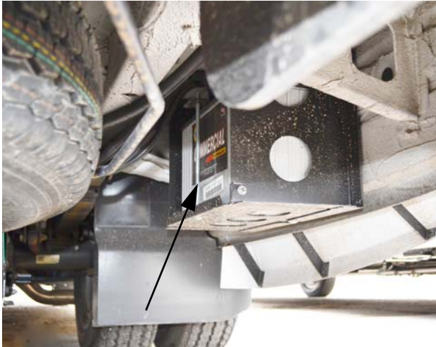
House Battery Access
