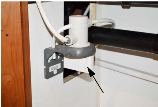
Diverter Plug (installed in filter socket)
