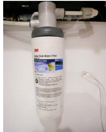
Cold Water Filter Assembly (Located inside lower galley cabinet)
