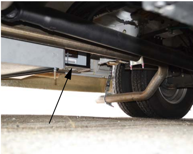
House Battery Access
