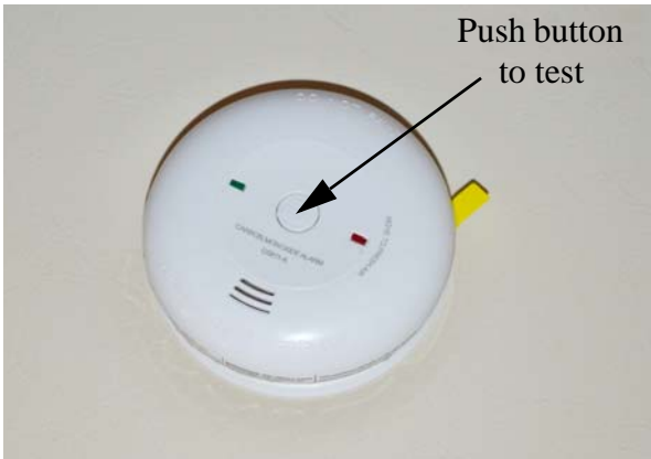
Carbon Monoxide Alarm
