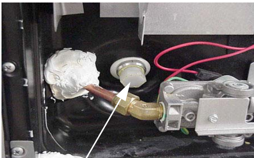
Water Heater Drain Plug (Remove with socket)
