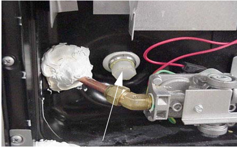
Water Heater Drain Plug (Remove with socket)
