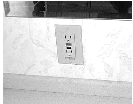
Ground Fault Circuit Interrupter (GFCI)
