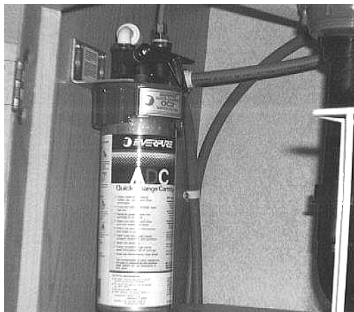
Water Filter Assembly - Below Galley Sink
