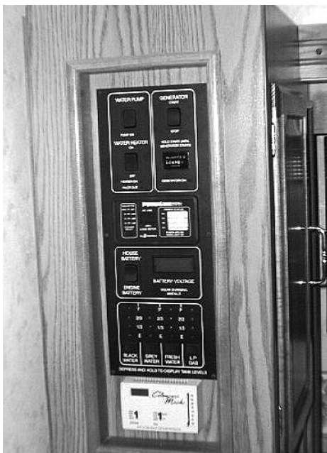
One Place Monitor Panel
