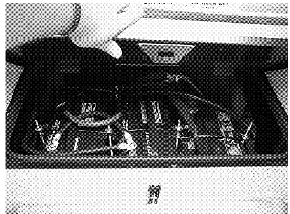
Lift step to access batteries
