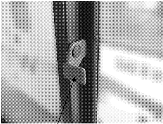
Lift Latch to Open Window (Be sure handle is also raised when closing)
