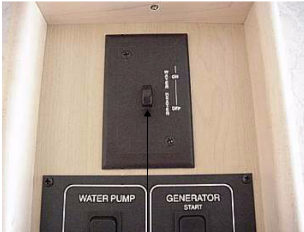
Electric Water Heater Switch above microwave oven Models 32V, 35U & 37G
