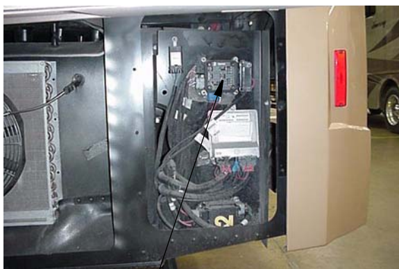
Towing Package fuses are on fuse block
