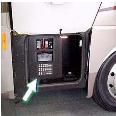
12V Electrical Compartment
